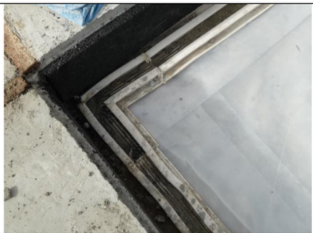
Separate Casting of PVC Waterstop
